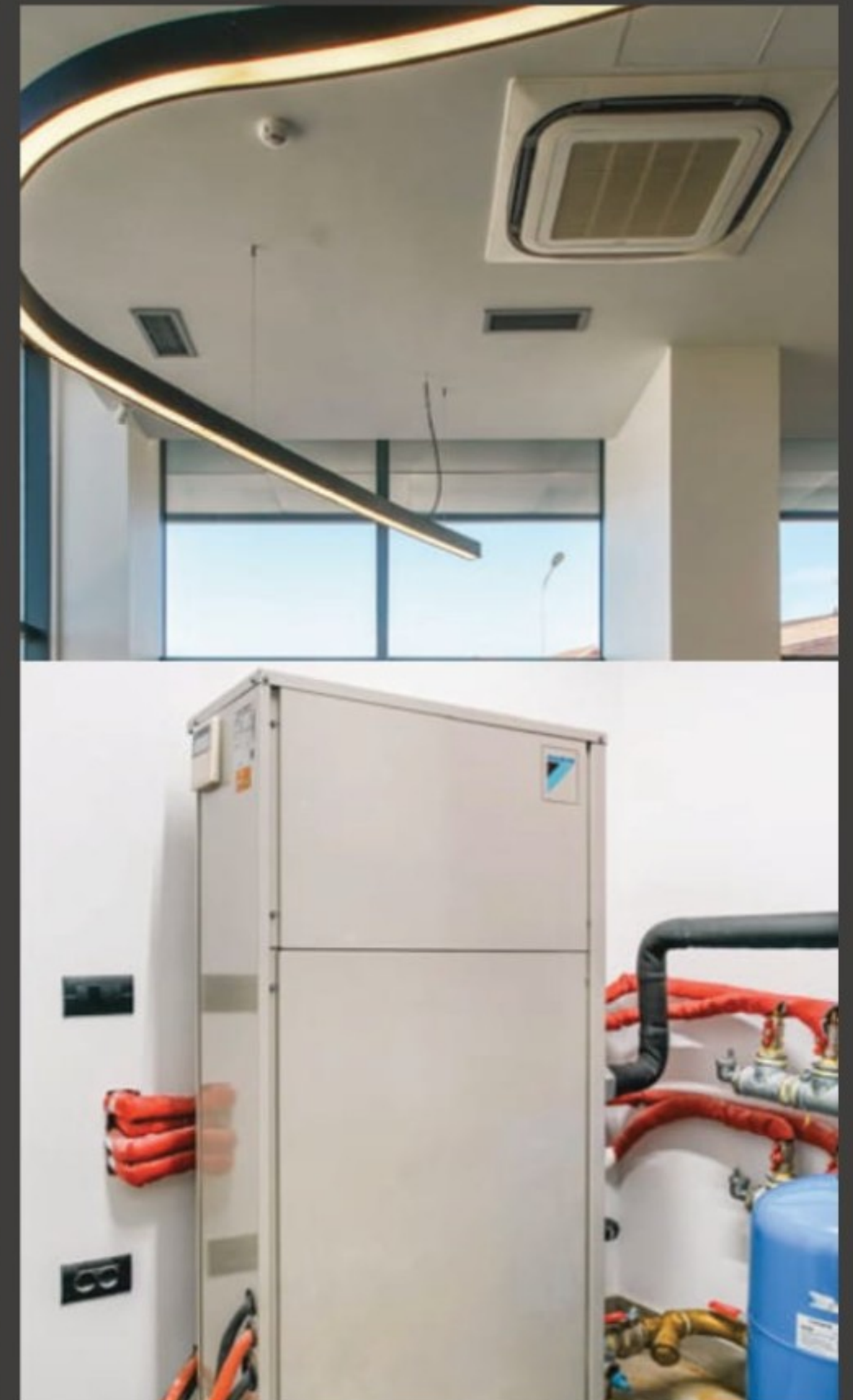
ILLYRIA INSURANCE COMPANY Prishtina 2021 Commercial object 700 m2 System installed: Daikin Underfloor Heating VAM Heat Recovery Units Daikin Altherma Flex HT HW Heat Pump Convectors
